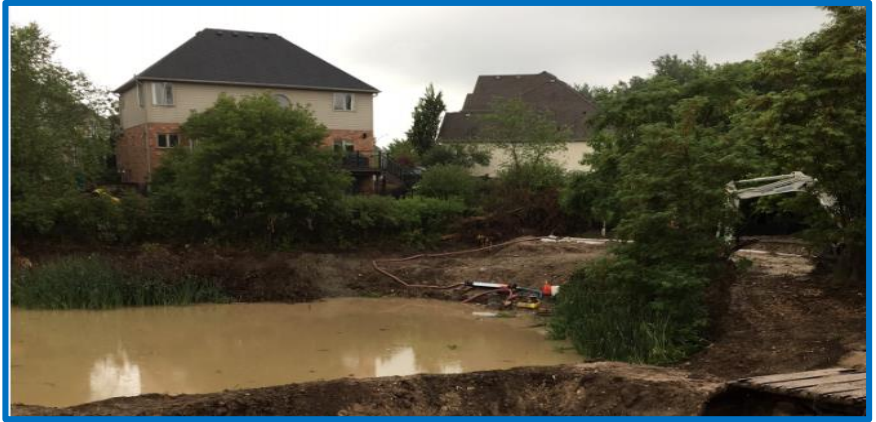
STORM POND SEDIMENTATION
